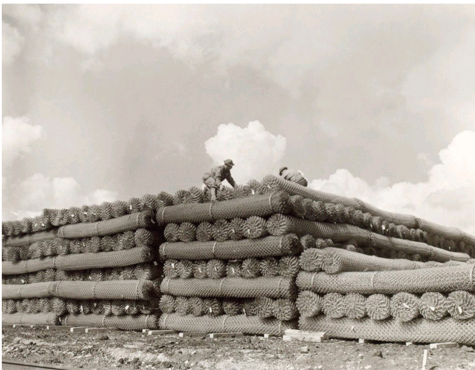
U.S. Army soldiers stack bundles of Square Mesh Track (SMT) that will be used as a surfacing material in the construction of advanced landing grounds in France after the invasion. National Archives and Records Administration/US Army Signal Corps 111-SC-189363
