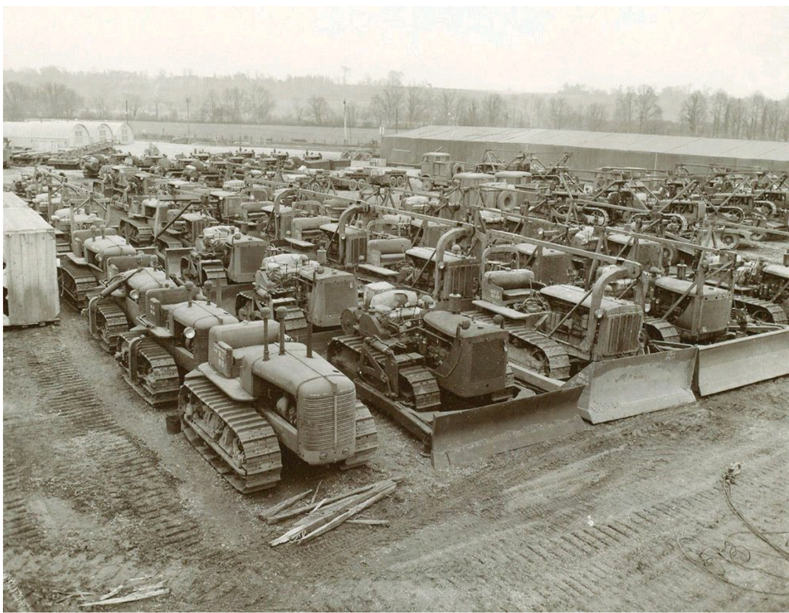
This view of the engineer depot at Thatcham, Berkshire, shows some of the different types of construction vehicles being amassed in England prior to the invasion. Here, Allis-Chalmers HD10W tractors, Caterpillar D4 tractors, and Caterpillar D7 bulldozers can be seen parked together in anticipation of the journey toward Germany. National Archives and Records Administration/US Army Signal Corps 111-SC-189366
