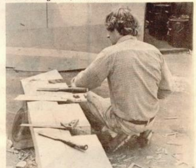
A SELECTION OF WOODWORKING TOOLS are unknowingly displayed to a casual onlooker as this worker chisels notches into the beam.
