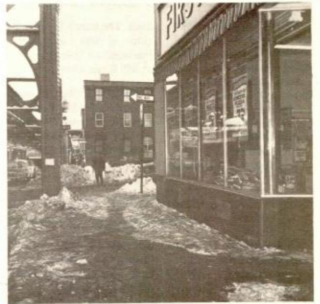
RESIDENTS were concerned about the pedestrian hazards that resulted when the management of the First National store at the corner of Main and Green streets failed to clear the sidewalks following a January 1968 snowstorm. The market is now the Charlestown Professional Building. The theater on the opposite corner had been razed, and the site would become the home of the Charlestown Branch Library.
