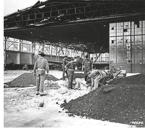
US Army airmen assess bomb damage at hangars on Hickam Field. ☹
