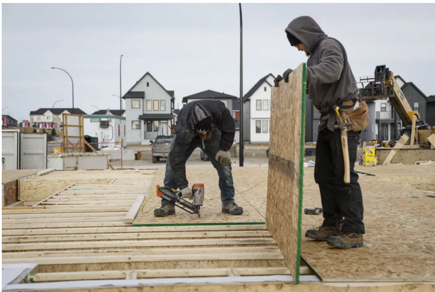
Framers work on a house under construction in Airdrie, Alta.
