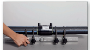
Clamps pipe and align it.
