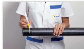
Mark the insertion depth.
