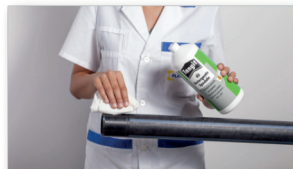
Clean the surfaces with a suitable detergent.
