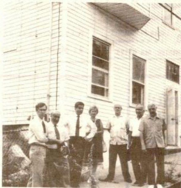
CITY OFFICIALS and neighbors of the abandoned house at 43 Belmont St. review their findings following a tour of the dilapidated structure. Shown (l. to r.) Peter Welsh, Inspectional Services Department executive director; Sonny Buttiglieri, ISD Housing Division supervisor; City Councillor Robert Travaglini; Judy Evers, community liaison, Mayor's Office of Neighborhood Services; John Hart, neighbor; Peter Bruno, ISD Housing Division inspector; and Frank Saccardo, neighbor. (photo by Kathy Giordano)
