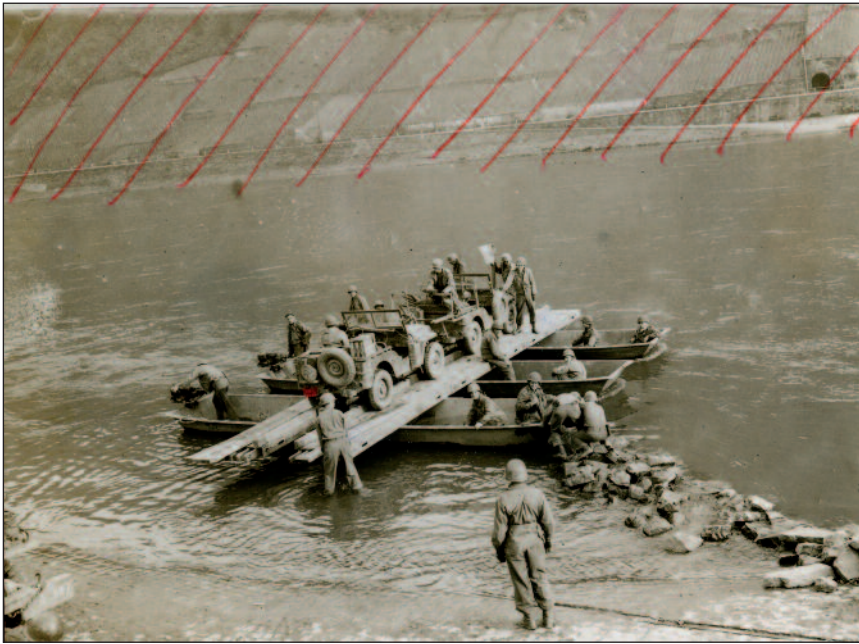
Two Jeeps being ferried across on a light support raft built by the division's 35th Engineer Combat Battalion.
