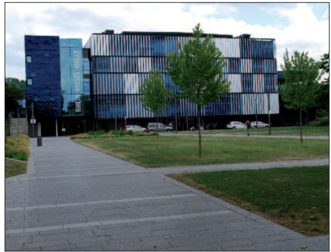
The Stadthalle stood at Am Mainzer Tor. Pulled down after the war, it was replaced by the Rhein-Mosel-Halle, erected in 1959-62 some distance to the rear of where the old building stood.
