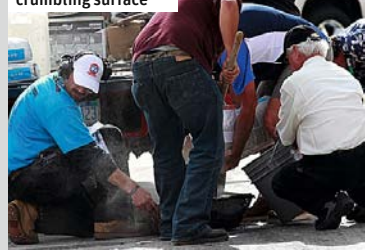
Track crew patch the crumbling surface
