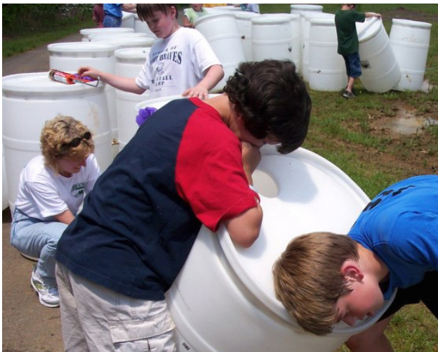
Students at Armuchee Elementary construct water barrels from donated soft drink barrels.
