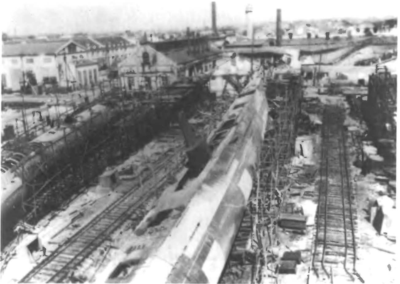
The Marti (south) yard at Nikolayev, like most of the southern USSR, was overrun by German armies in 1941. This view of the yard shows the unfinished S-37 (left) and S-36 still on the building ways. Other incomplete submarines as well as surface ships were towed to Soviet-held ports farther east for completion. (German Army)
