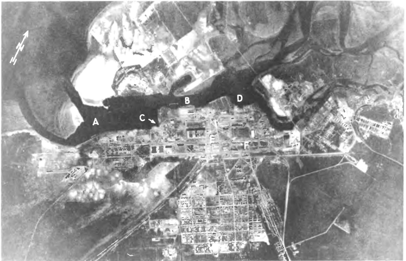
The primitive facilities of the Molotovsk Shipyard at Severodvinsk were vital to the fitting out and maintenance of Northern Fleet submarines. The yard was photographed by a German aircraft in July 1941: (A) naval base; (B) fitting out area; (C) dry dock with entry locks under construction; (D) wharf; (E) construction hall No. 42; and (F) metal working plant. ( Luftwaffe photo)
