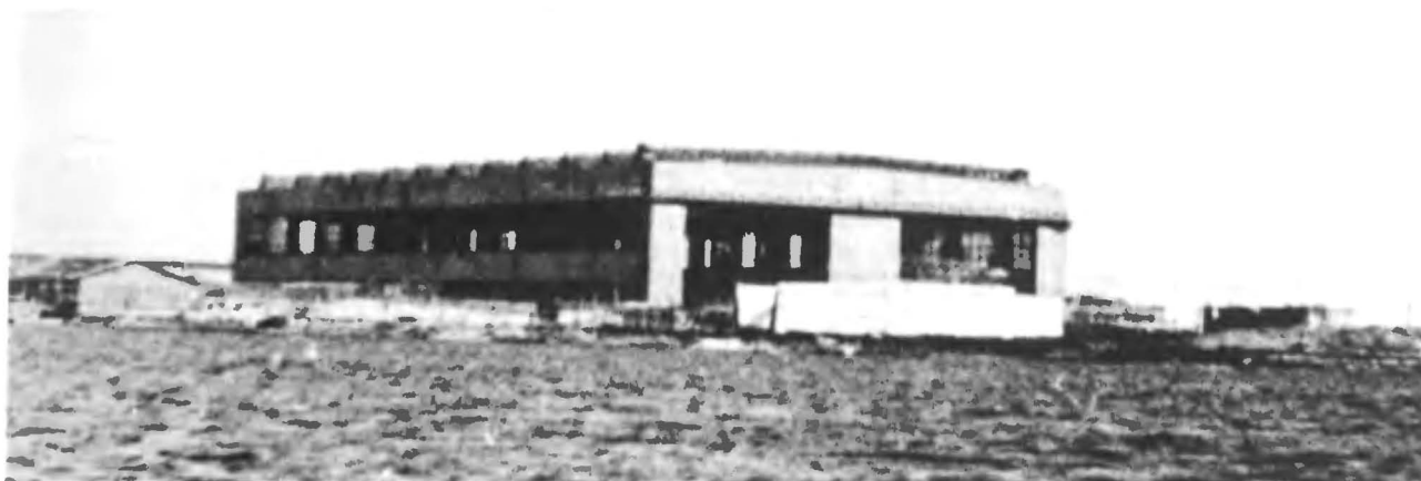
Building hall No. 42 at Severodvinsk was erected on Stalin's orders to construct major warships for the Northern Fleet. The facility—shown here in June 1944—was intended to construct two battleships simultaneously. It is now part of the world's largest submarine construction yard. (U.S. Navy)
