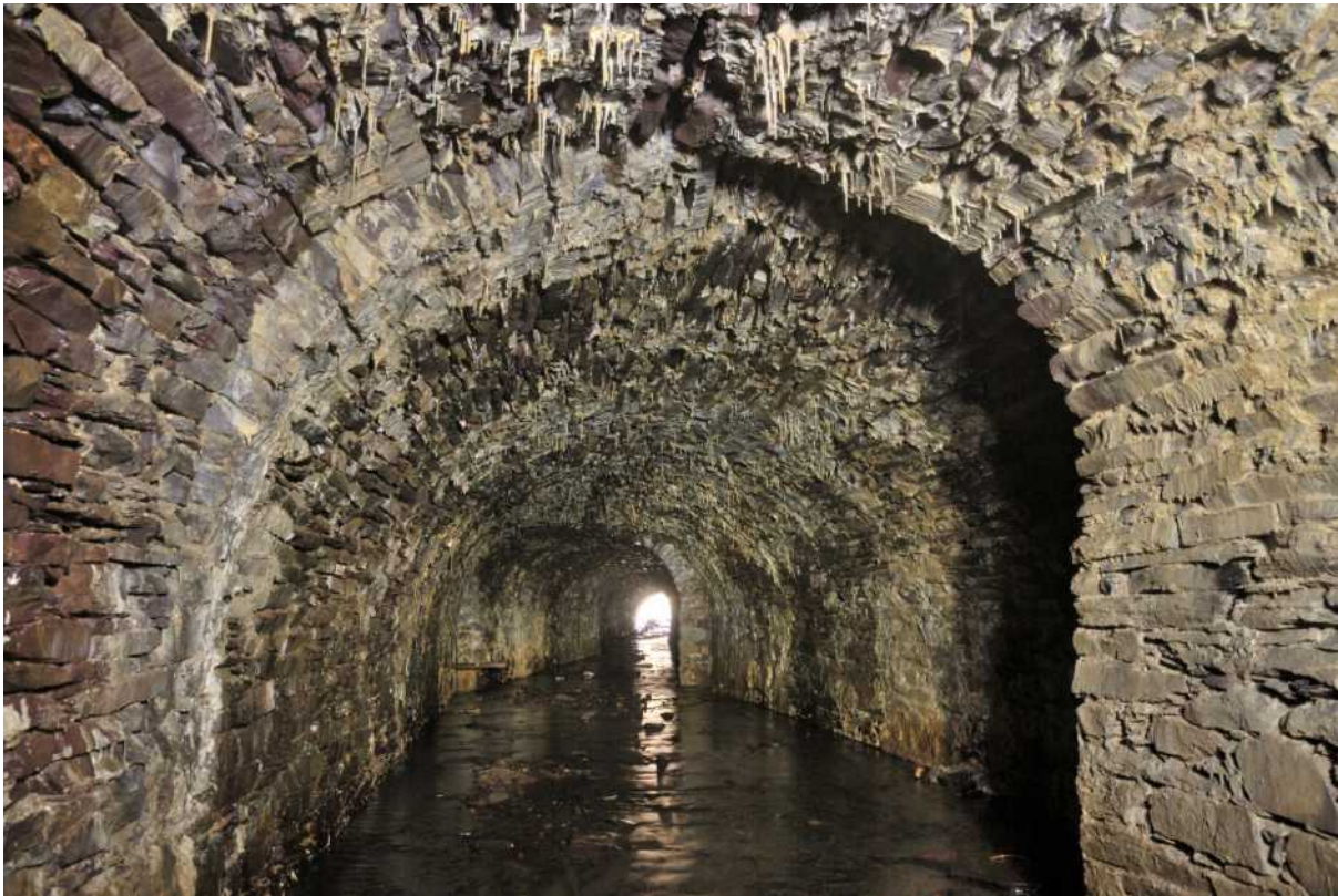
11. Looking east from ~85 metres inside the tunnel from the eastern portal, showing interfaces and change in alignments between tunnel sections. It is not known why it was built in sections, rather than as a continuous structure. The section shifted to the right seems to have been built to fill between the sections in the fore and background.
