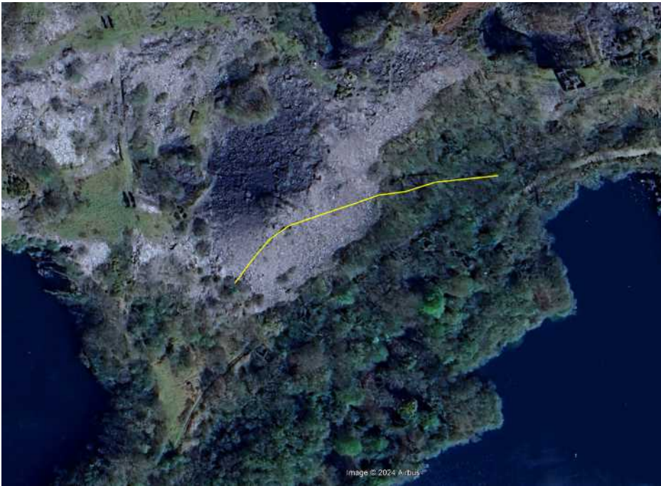
5. A more detailed view of the Blaen y Cae tip and full tunnel length plotted against the surface view. The western access to the tunnel is tantalisingly close to the edge of the tip's final extent. Because the western end was a busy incline landing area, this adds to the impression that tipping from Talysarn quarry (at extreme left) was unlikely to have taken place here or over the tunnel, though frequent changes to these constrained quarry sites make definitive conclusions difficult.
