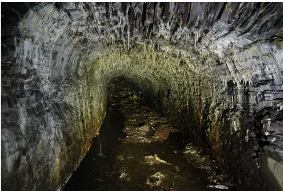
13. Western, blocked extremity of the tunnel, considered to be the natural built end, rather than a collapse. Slate blocks part way to the roof may have been deliberately set, but this is unclear. Waste within the tip is clearly visible as clean slate beyond. The tip edge and open air is probably only a few metres away. The culvert portal (see 14) emerges just in front of the blocking slate, on the right. The round rampant arch profile is very clear here.
