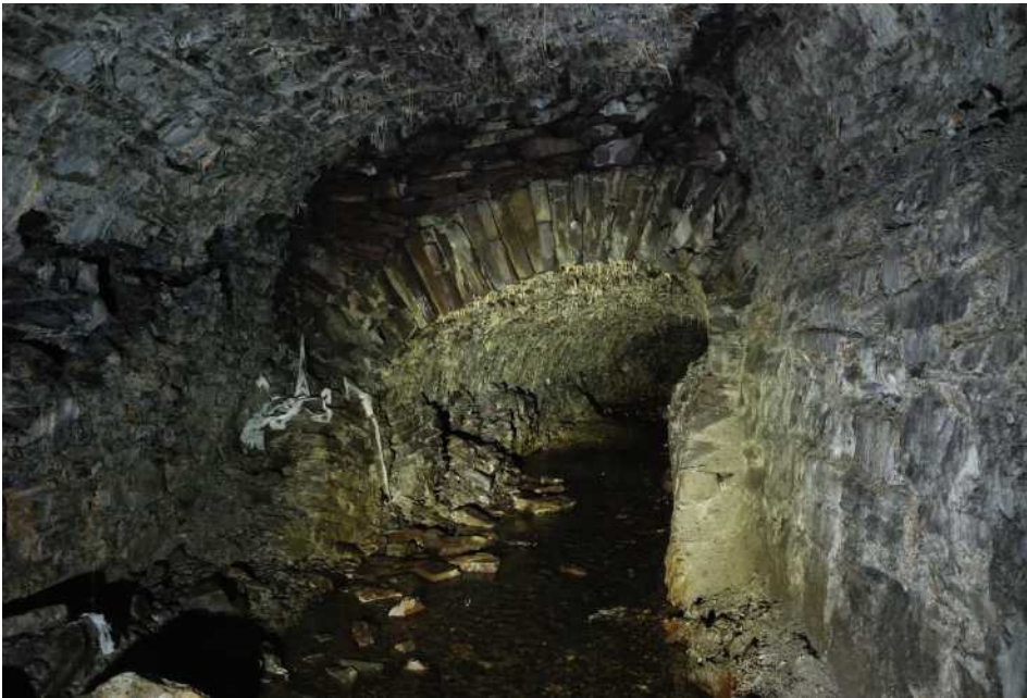
12. Looking back upstream in the tunnel (towards the eastern end) with a secondary reinforcing arch and packing above (camera at ~130m in). Low buttressing to ~1.2m up is seen along the northern (left) wall. The left face of the secondary arch and surroundings are missing blocks and slowly working their way to what would likely be a catastrophic collapse. There is room only for one track and only one was mapped as emerging in 1889. The white material at left is 'geocaching' decoration – the most ridiculous reason of all to place oneself at very high risk by being present anywhere near this section.
