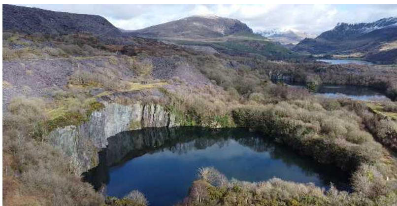
3. View of Talysarn quarry pit, now flooded and Dorothea, glimpsed at centre right. The tunnel runs under the tip at upper centre. Photo: 2024 March 03.
