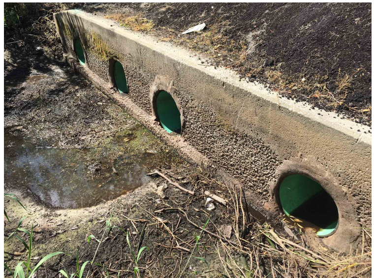
Figure 4: Existing Pipe Culvert (2017 drought)
