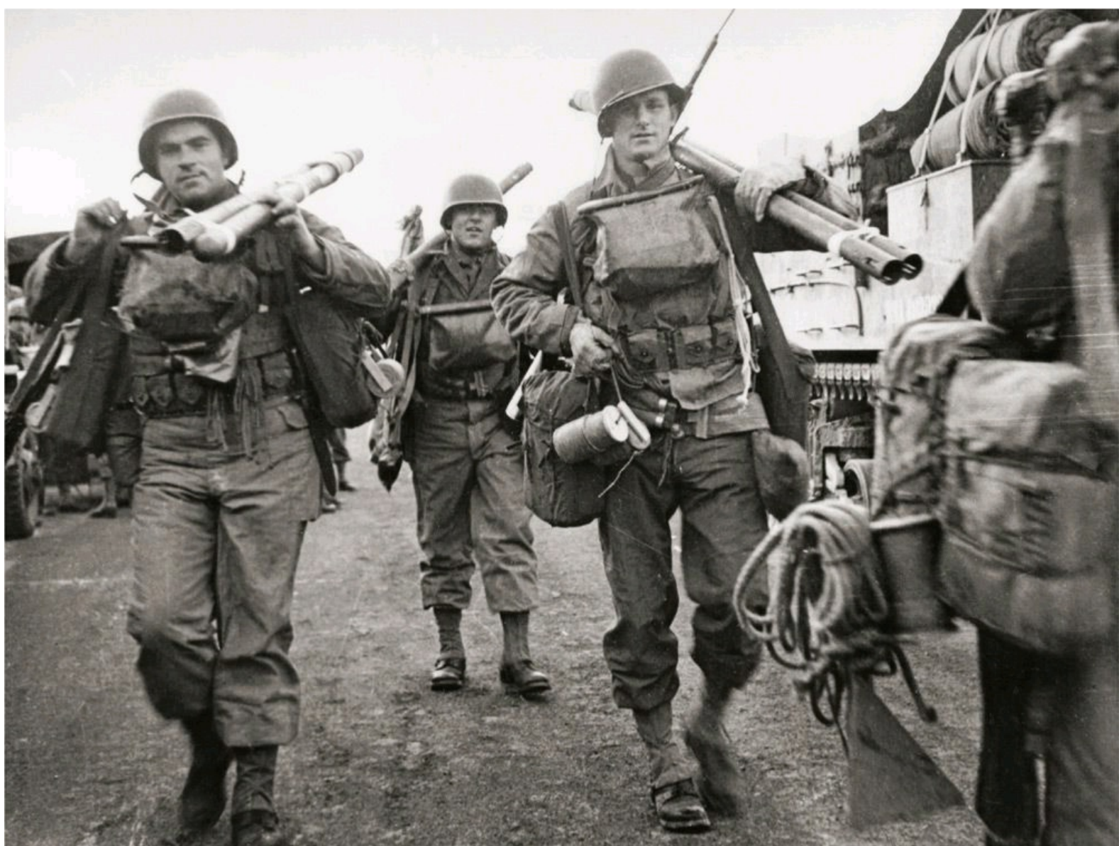
Three U.S. Army combat engineers from either the Special Engineer Task Force or Beach Obstacle Demolition Party move to their embarkation assembly area in preparation for D-Day. Each soldier carries a section of Bangalore torpedo on his shoulder, reels of Primacord, and an M7 Assault Gas Mask Bag worn on his chest. The man in the center already has his M1 Garand rifle packed in a Pliofilm bag to protect it from sand during the landing. National Archives and Records Administration
