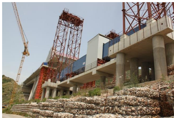
Figure 18. Piers of the right branch
