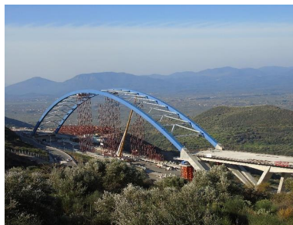
Figure 11. Removal of the towers
