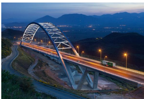
Figure 33. The completed Tsakona bridge
