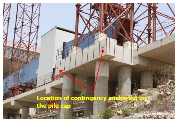
Figure 32. Prediction of anchoring of the pile-caps
