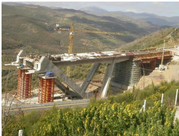
Figure 8. Construction of the prestressed concrete part of the bridge deck
