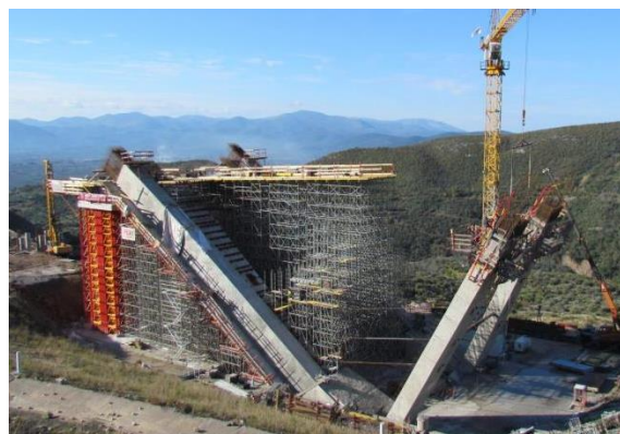
Figure 6. Construction of the pier struts
