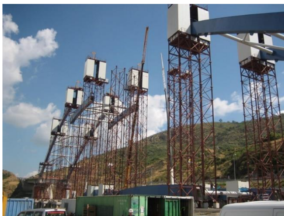
Figure 9. Assembly, erection and welding of the arch segments
