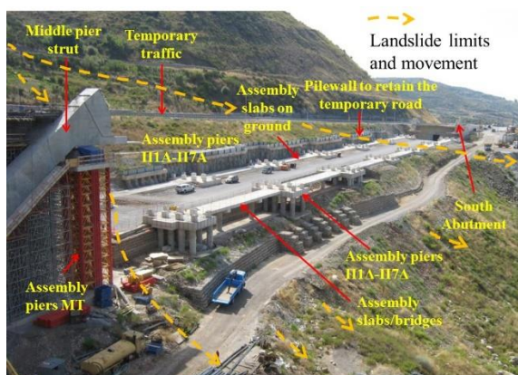
Figure 5. General view of the worksite
