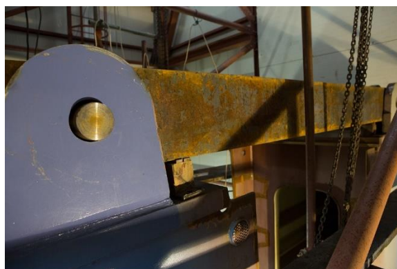
Figure 10. Fixing the gap between the arch parts to weld its last piece
