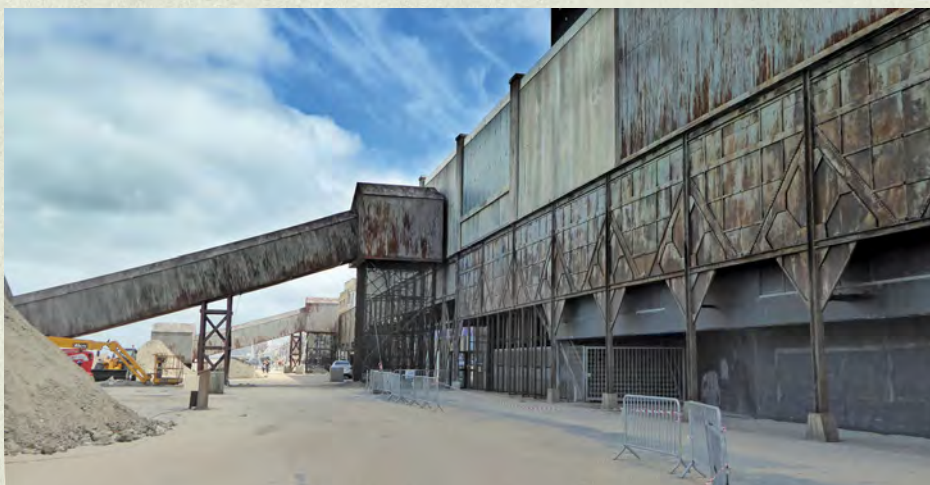
ABOVE: The Kursaal very convincingly disguised as a pre-war factory. Even close up the disguise appears very authentic. The cladding is largely plywood, painted to represent rusting steelwork. Some modern ISO containers are incorporated too.
