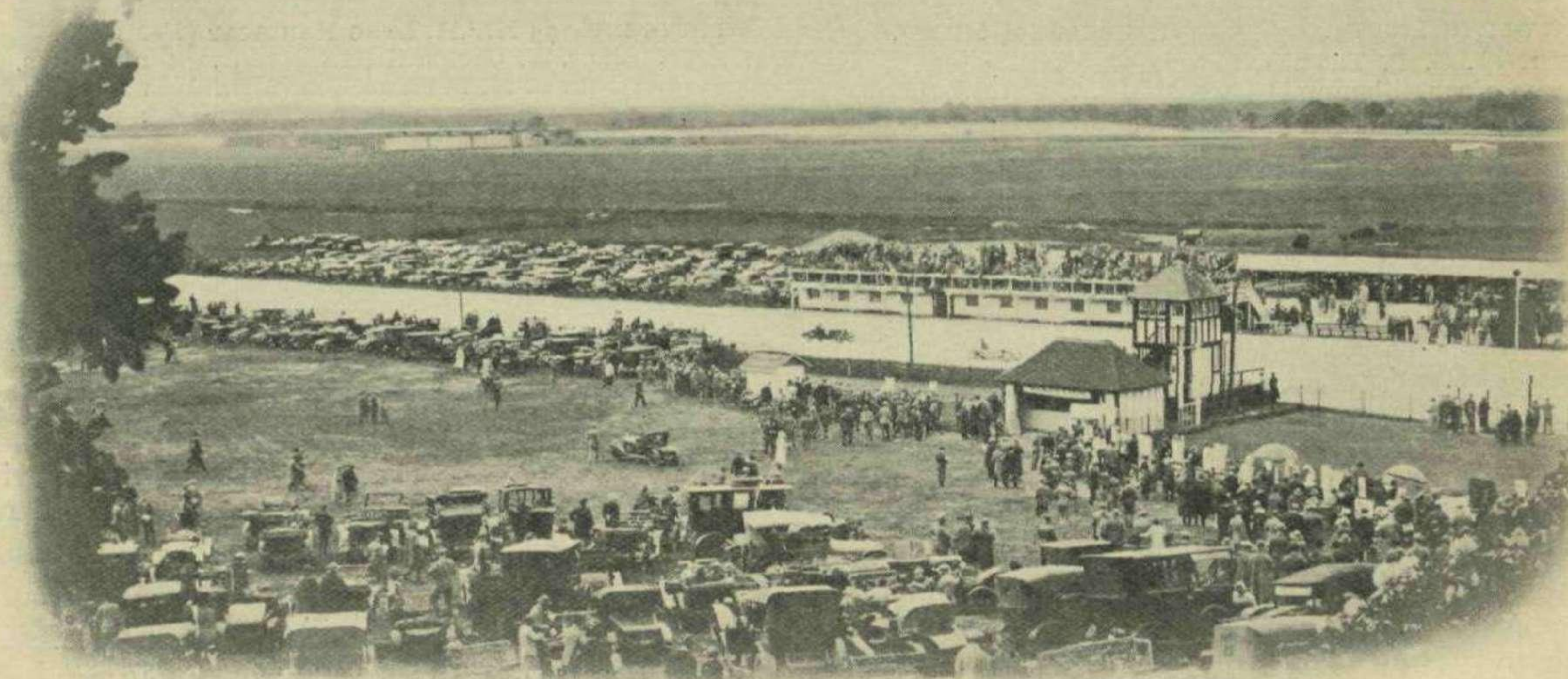
A VIEW FROM THE TEST HILL.
