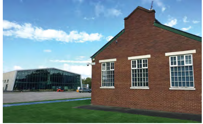
ABOVE: More will be made of the surviving 1931 buildings at Hendon, while the former Battle of Britain Hall (left) becomes the museum's new 'introductory' exhibition on 100 years of the RAF. BEN DUNNELL
