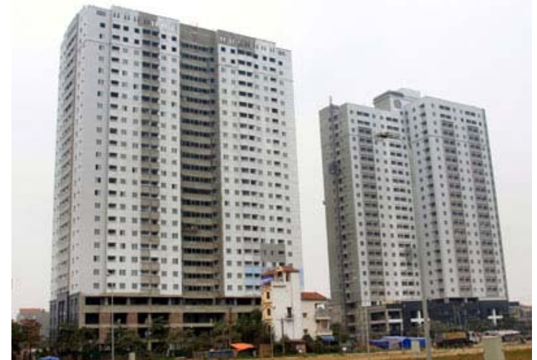
CT1, CT2 NGÔ THI NHẠM/ CT1, CT2 NGO THI NHAM BUILDING
