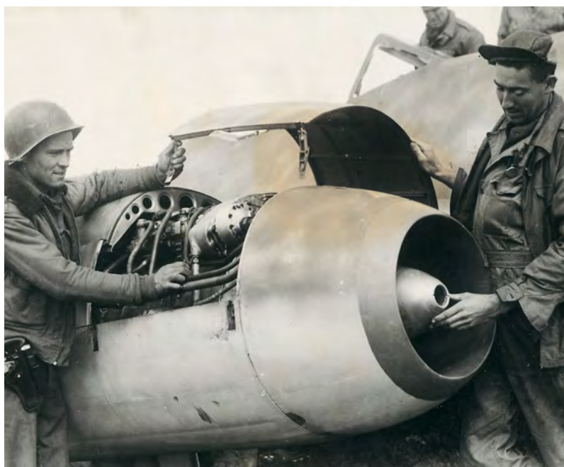
US personnel examine one of the Junkers Jumo powerplants on a captured Me 262.
