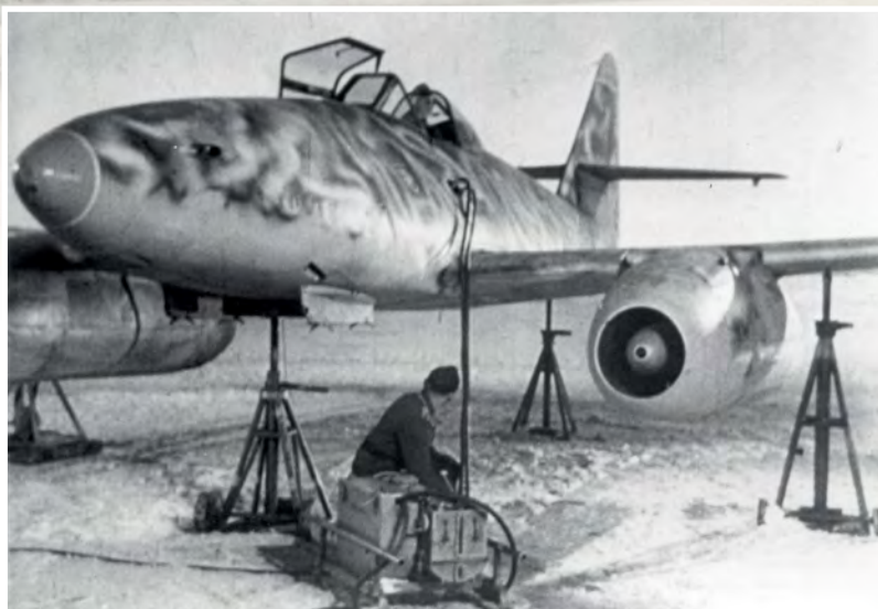
A Messerschmitt Me 262A-2a undergoes wheel retraction tests.
