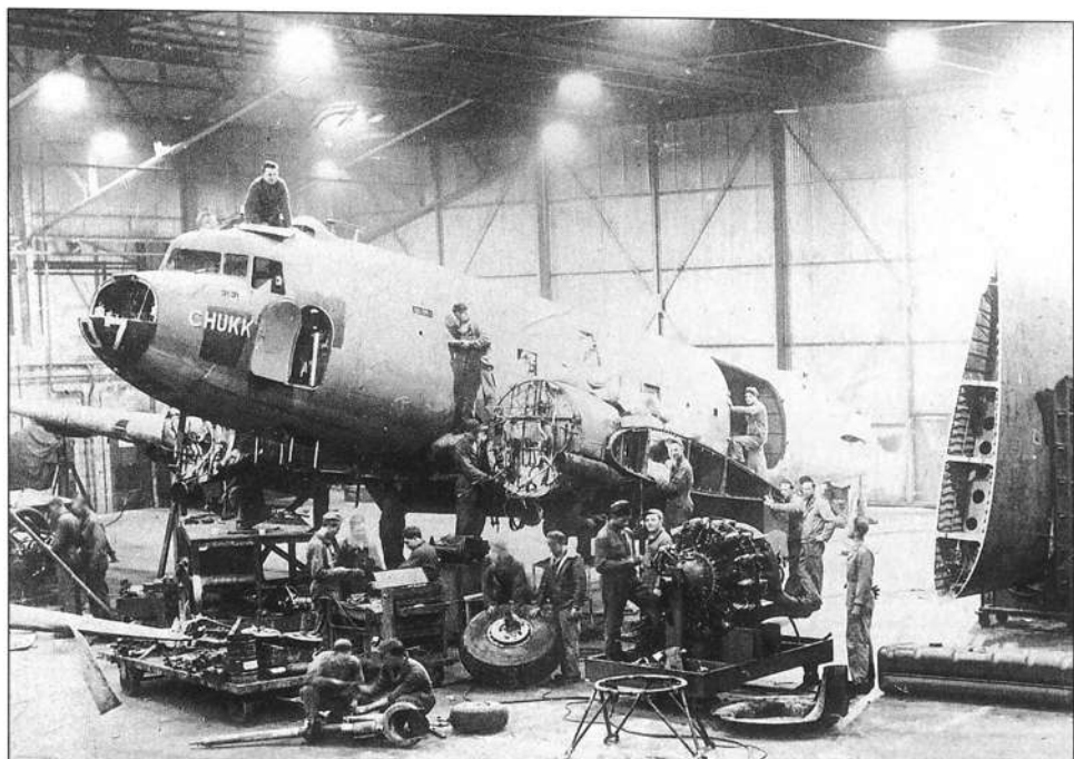
A C-47 being completed overhauled by engineers at BAD 2 (Base Air Depot), at Warton, near Liverpool, England, during the Second World War.
