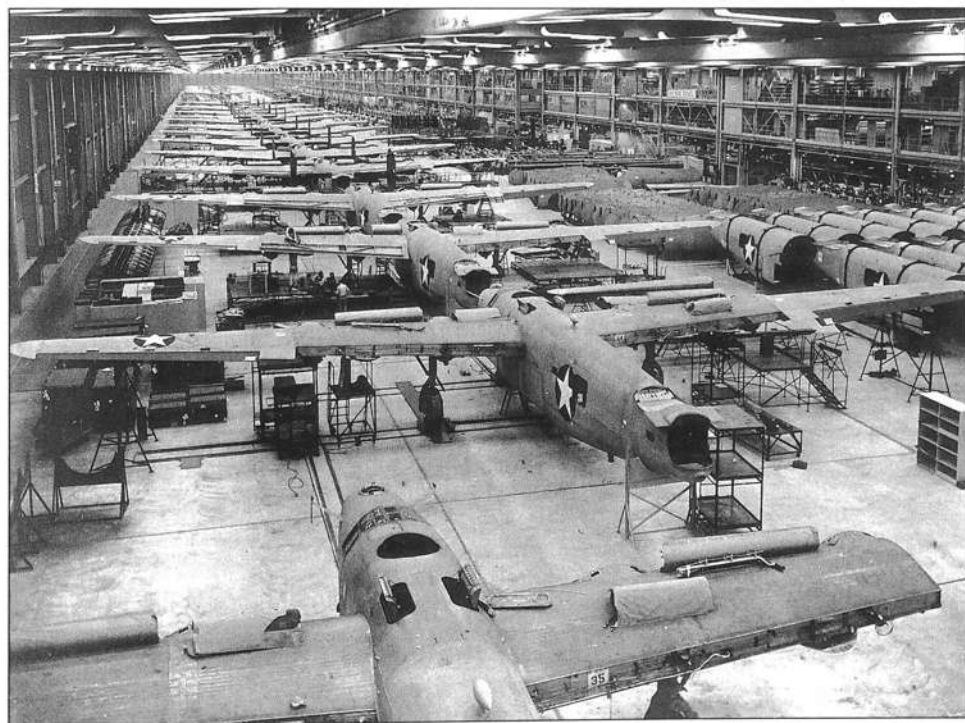
A third B-24 Liberator production line was brought into operation at the Tulsa, Oklahoma plant in March 1943.
