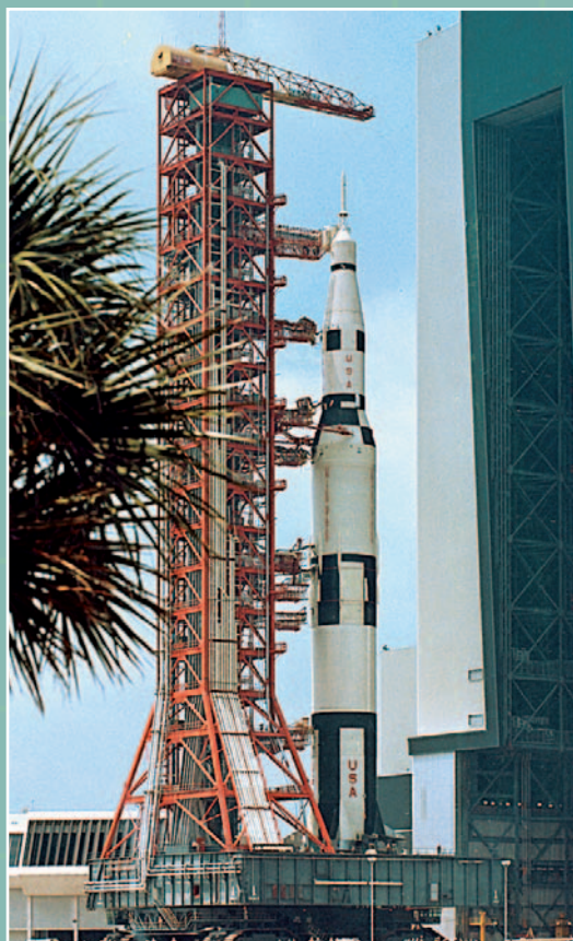
The stages of the giant Saturn V rocket were stacked together inside the enormous Vehicle Assembly Building (VAB), one of the largest buildings ever constructed. Here, the Saturn V is being moved from the VAB (located at the Kennedy Space Center in Florida) to its launch site.
