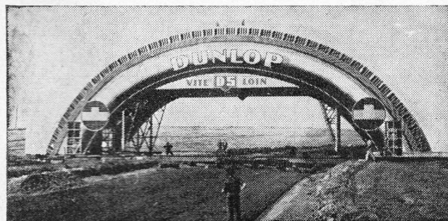
LE MANS, LATEST: Work proceeds apace on the new pits and circuit alterations at Le Mans, in readiness for the G.P. d'Endurance on 28th-29th July. (Left) The 30-ton Dunlop bridge beyond the pits was removed bodily on rails to its new site.
