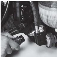
(2) Determine which cylinder retainer kit is needed (if you already have existing MSA cylinders). New cylinders with retainer kits already installed are available for purchase. Contact the local MSA Sales Manager or local distributor for more information and part numbers.
