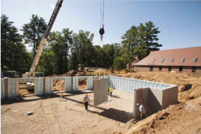
Superior Walls Avon Old Farms School – Poirier Homes
