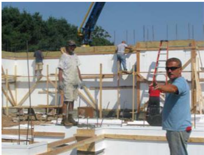
Joe Ciarleglio directing construction.
