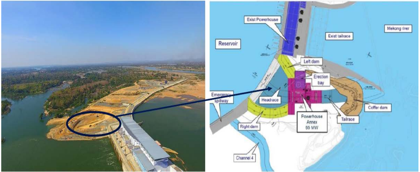
Figure 1: 5 th Turbine Construction Progress as of end-May 2022 (65MW)
