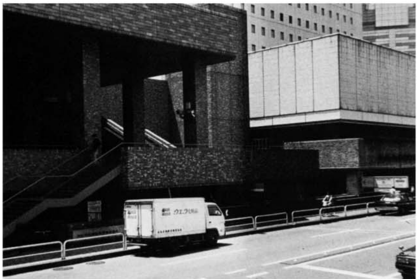
A present day visitor can still sleep on the site of the cell blocks — if one books into the Prince Hotel!
