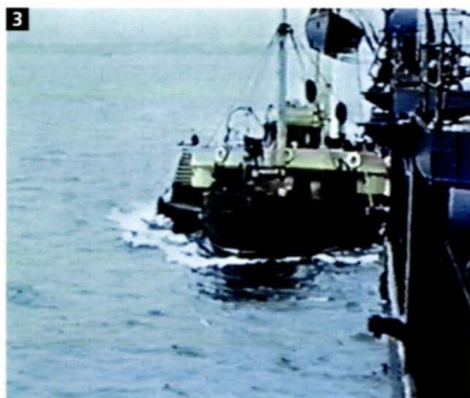
3 An Admiralty tug helps the Hood out of Portsmouth in the summer of 1939. Starboard No. 3 5.5in gun is visible on the right.
