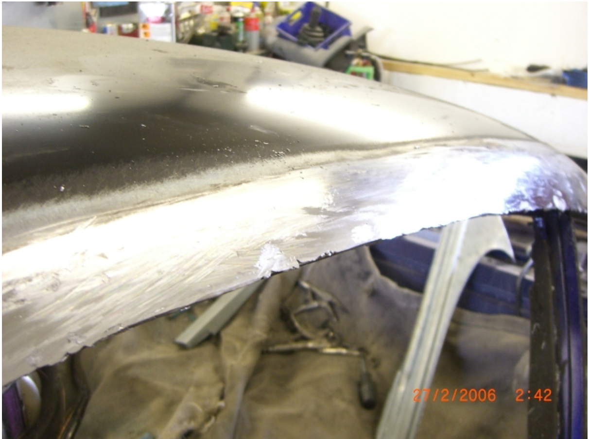
Gutters removed and leaded.
