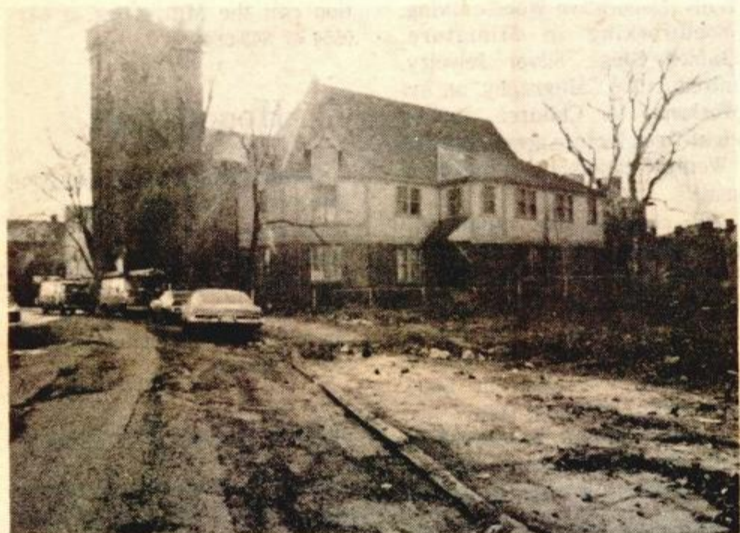
RUBBLE covers the sidewalks of Devens Street and numerous potholes in the area of senior citizen apartments on Devens Street and Old Rutherford Avenue are hazards that the Charlestown elderly must face daily. (photo by Bill Winder)
