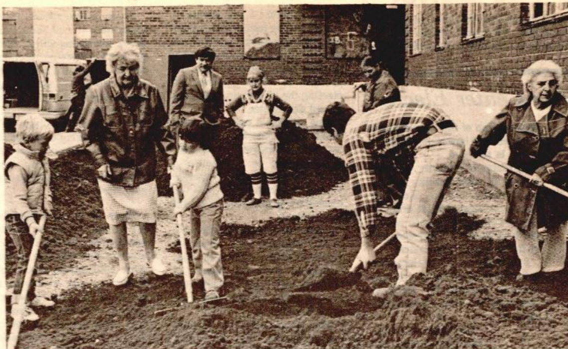
LOAM DELIVERED: Boston Parks and Recreation Commissioner John Vitagliano, left, with Mrs. Edna Boyle (Mrs. Bee) discuss the work done by residents at the Bunker Hill Housing Project, during delivery of loam by the City. Tenants of all ages, in front, are shown working on the landscaping.
