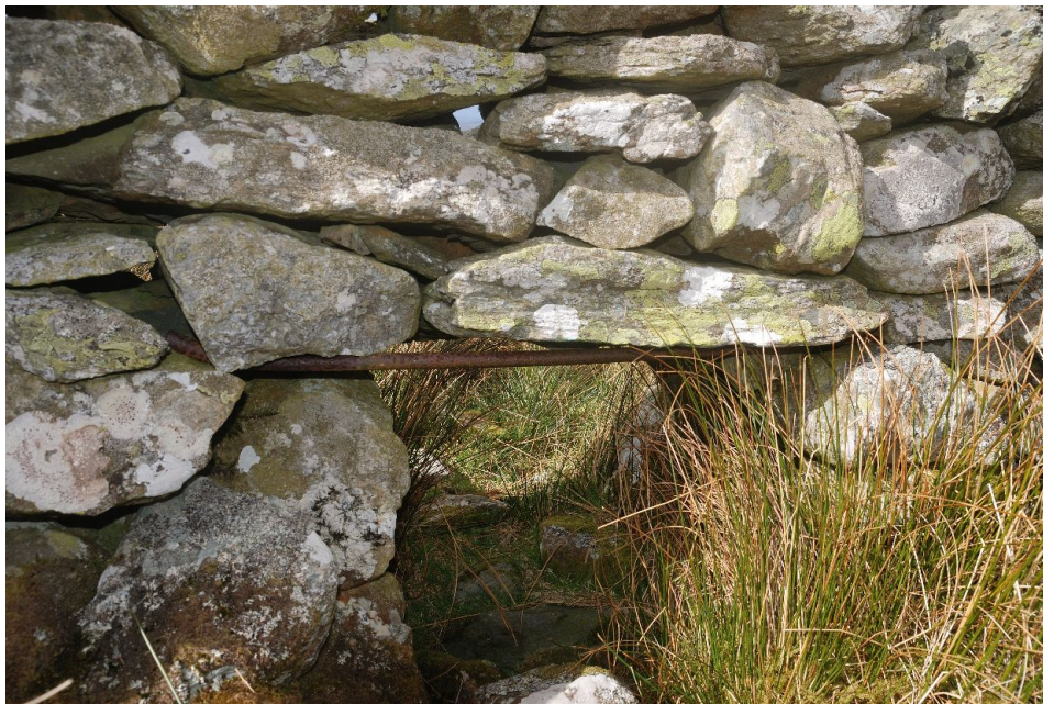
Iron bar part-lintel over an outer cell creep hole at Afon Llafar fold, NPRN 24404.
