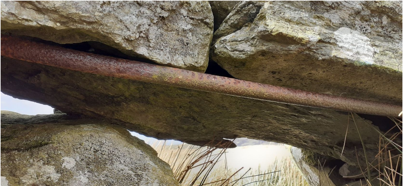
Underside detail of iron bar part-lintel, showing its use over a limited part of the creep hole opening.
