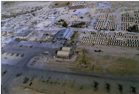
An aerial view of Kandahar air base from the front seat of an AH-64. Chinooks, Blackhawks and Apaches are visible in this photograph. The tent city in the upper right hand corner of the shot is the pilot and groundcrew living area (CW4 Zac Noble)
