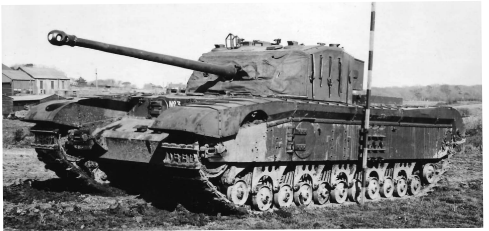
Black Prince number 3 with a measuring post alongside. From this angle you can see how the track guards sloped down at the front, ostensibly to improve the driver's view.
