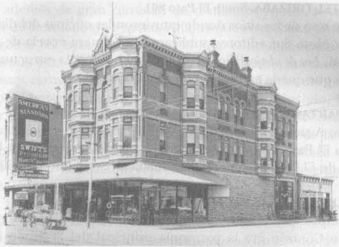
Edificio Merrick (Shelton-Payne Arms Company), ca. 1913. (Aultman Collection, El Paso Public Library)
