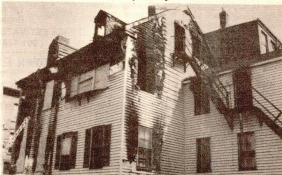
A TWO-ALARM FIRE early Saturday morning destroyed this two-family house at 21 Oak Street. The occupants were able to escape safely from the building.
