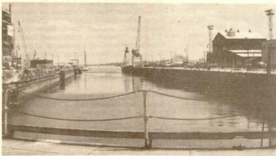
DRY DOCK 2, as seen from First Avenue at Gate 4 with Shipyard Park on the left and Pier 3 on the right. On Wednesday, May 10, the Charlestown Neighborhood Council Aquarium Committee-of-the-whole, by a 14 to 5 vote, gave approval to the New England Aquarium to continue to develop a proposal for Dry Dock 2. (photo by Kathy Giordano)
