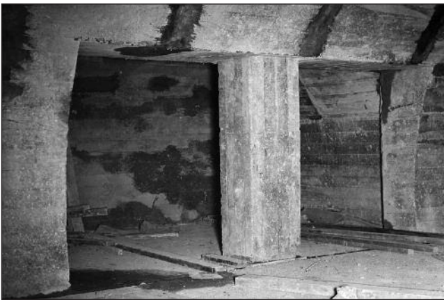
Left: These photos are part of a series taken by E. J. Wright on May 1, 1943, when the underground facilities were still under construction. This is the Battery Plotting Room, looking out to
