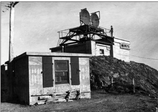
Left: The radar station at Moa Point below Palmer Head was set up in April 1942. The two lower buildings were for an imported Australian ShD (Shore Defence) Mk I set. The upper
