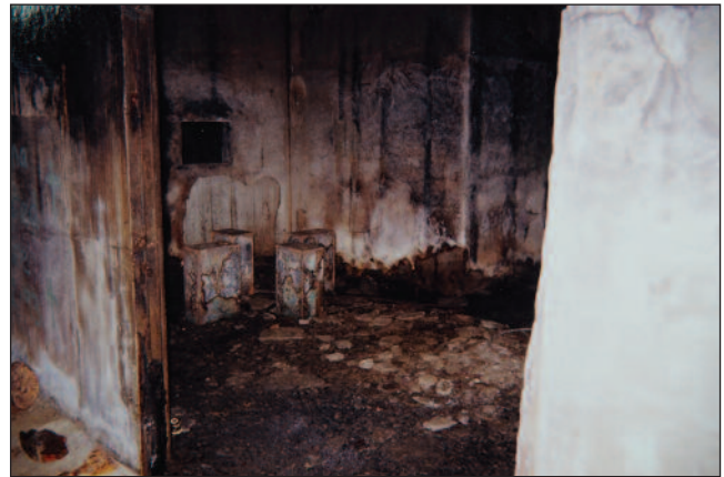
The underground installation was never fully operational due to leaks and Darcy found the L-shaped tunnel partially blocked and still flooded. This is the Battery Plotting Room, still featuring the pedestal for the coordinate converter. The hatch in the wall connects to the Fortress Plotting Room.
