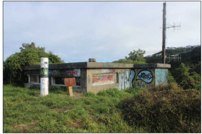
Another survivor is this radar post on the hillside above the Night BOP. It was added in November 1943 to house a British CD No. 1 Mk V set.
