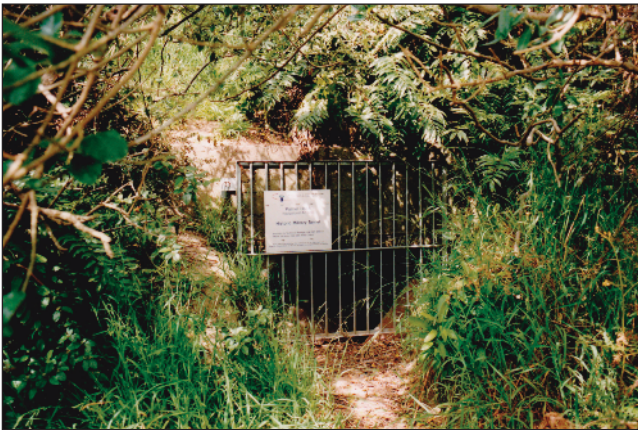
The battery's underground plotting rooms still exist but access to them is restricted due to the hill's current use by Airways New Zealand. These pictures were taken by Darcy Waters in 1998, who had to sign a safety disclaimer before he could borrow the key for the tunnel's access gate.
