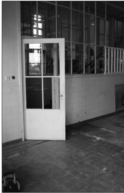
Entering the station's generator room, the men swung left, through a door . . .
