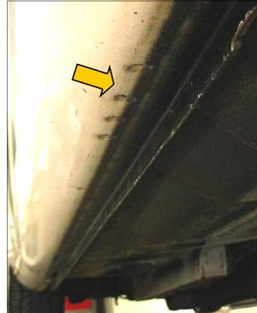
Rocker panel pinch weld black-out-often it is not this wide
