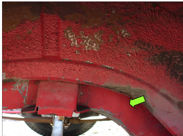
Paint worn from sound deadener in spots from use. Arrow shows nice exterior coat on frame rail
