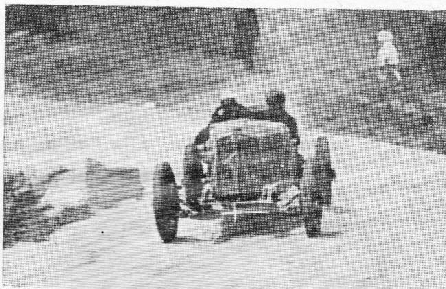
FIRST MAJOR WIN for Alfa Romeo came in 1923, when Ugo Sivocci won the Targa Florio in a 4½-litre six-cylinder push-rod o.h.v. car, similar to that shown.
