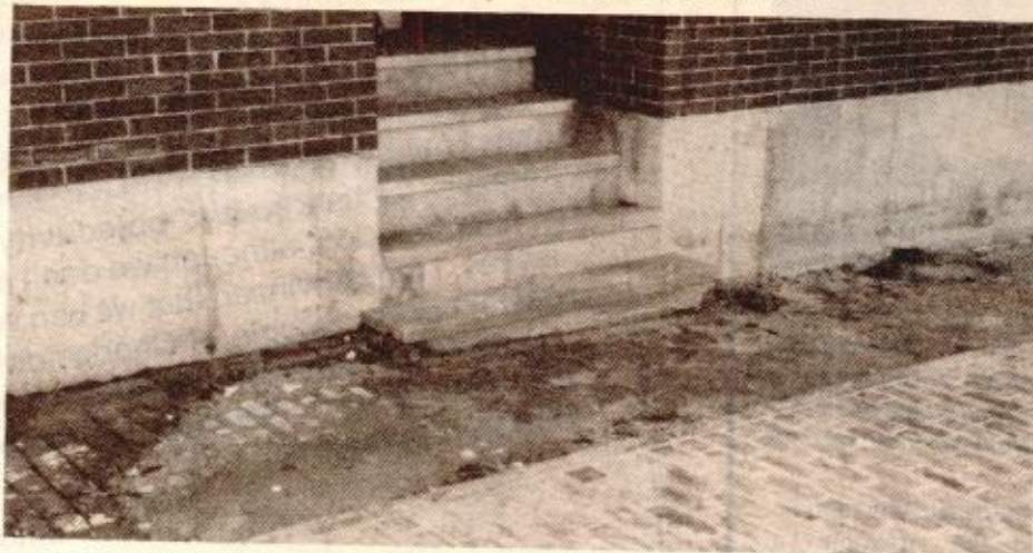
THOMPSON GREEN on Main Street may have a 30 foot sidewalk, but the brick side-walk does not meet the doorsteps or the foundation of the building.
