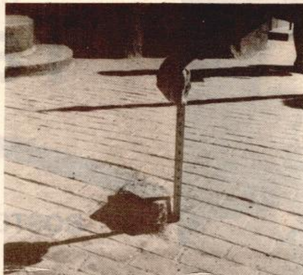
ONE OF THE survey location standards left protruding three inches above the newly laid brick sidewalks.
