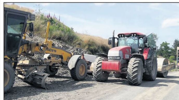
Rally4Wales firm has taken over the road repair job from NRW
