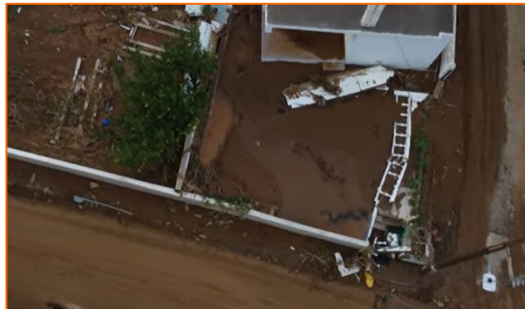
Yard walls and fences suffer structural damage (Photo credit by Prof. Dr. E. Lekkas and skai.gr)
