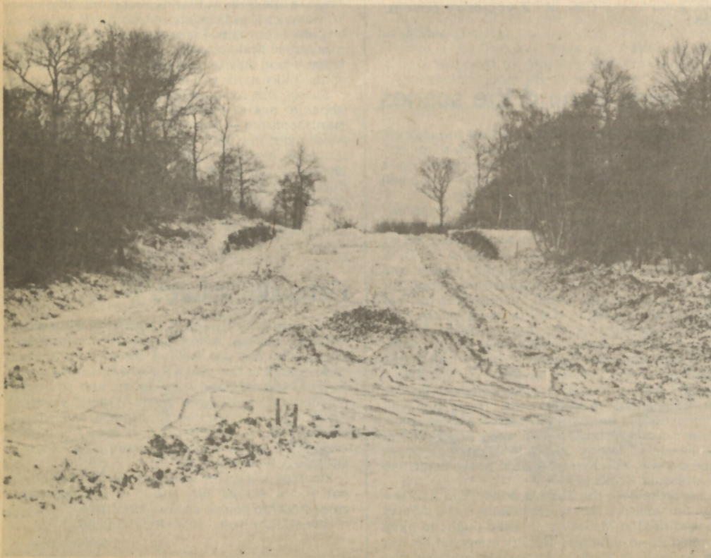
The Druids extension being built in 1954.
