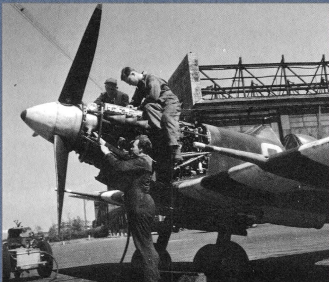
American and British mechanics work on a VCS-7 Mk Vb.
