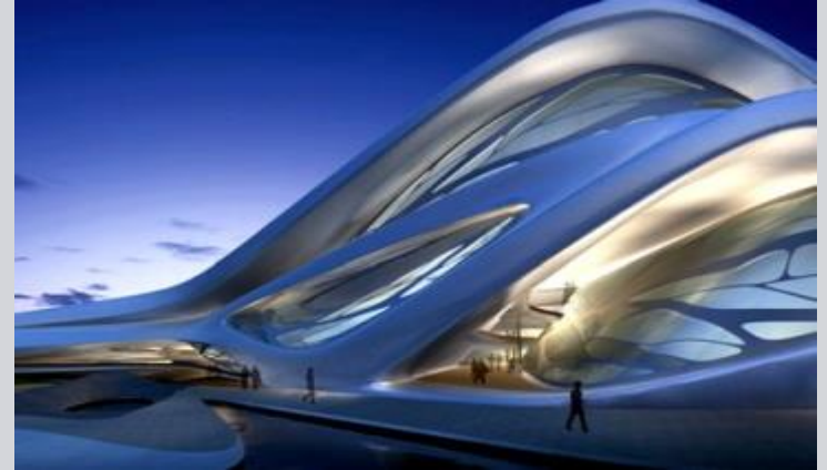
Performing Arts Centre Abu Dhabi
