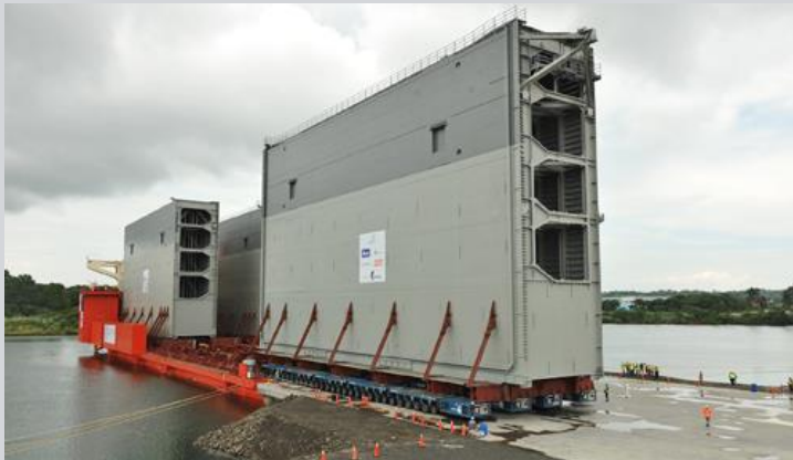
Steel gates of New Panama Canal
