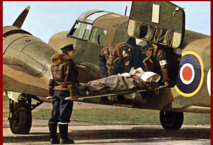
ABOVE: A staged shot of a 'wounded' airman being loaded into an Oxford by three nurses in flying kit shows the ambulance version's modified entry door. VIA JAMES KIGHTLY
