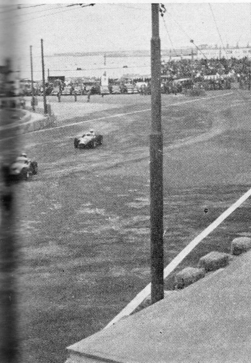
Evans and Shelby, over the tram- additional hazard.
