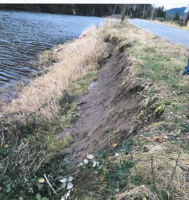
Figure A-3: Section of Seabird Island Road embankment sloughing - approximately 10 m long
