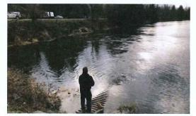
Figure 3-12: Surcharged culvert servicing private driveway
