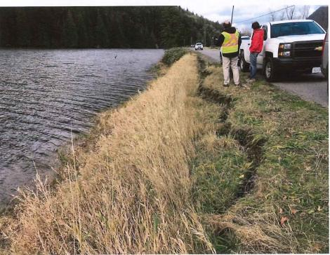
Figure A-1: Section of Seabird Island Road embankment sloughing - approximately 50 m long
